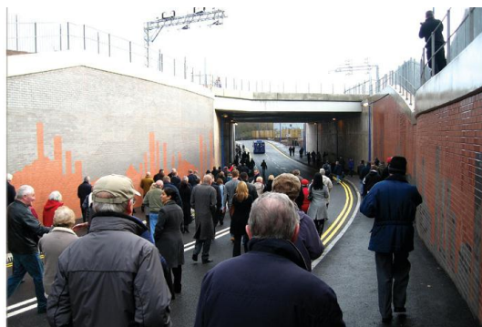
Photograph: The Owen Street Level Crossing at Tipton, 2010. (Proceedings of ICE Feb 2011, Paper 10-00025)
