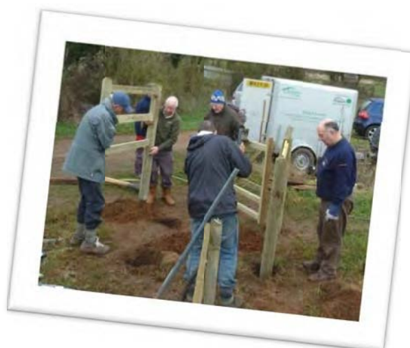
Volunteers installing gate ( Howard Dell)
